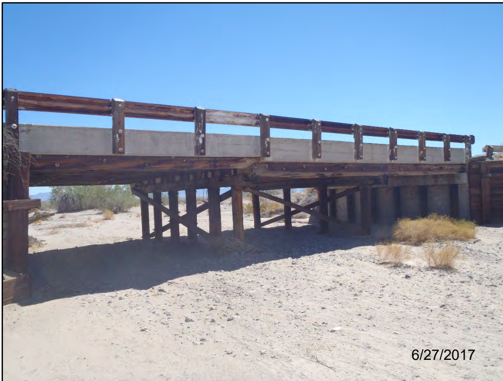
Photo 7. View of Sutro Ditch Bridge (#56C0104).
