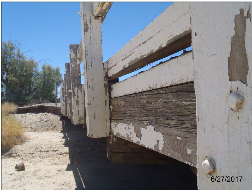
Photo 2. View of the timber bridge at Aztec Ditch (#56C0102).
