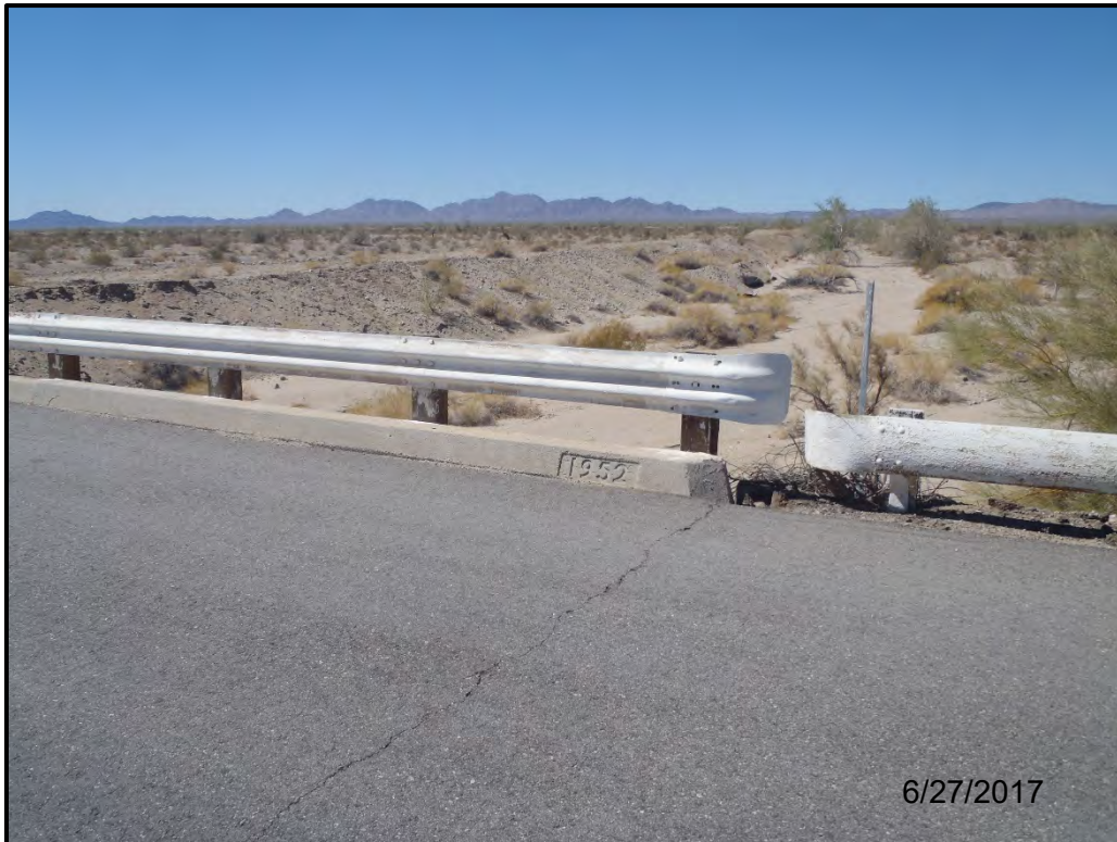
Photo 9. View downstream of the Acari Ditch Bridge (#56C0108).
