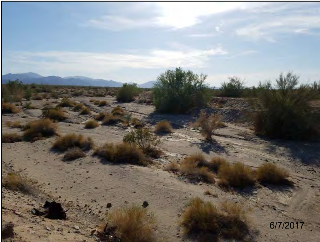
Photo 11. View of vegetated portions of the desert wash from Acari Ditch Bridge (#56C0108). Diversion dikes are present in and along the banks of the wash. Facing west.
