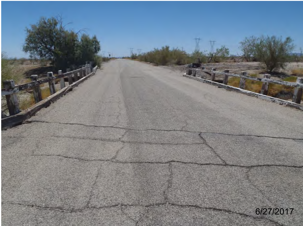
Photo 3. View of Chuckwalla Valley Road adjacent to Aztec Ditch Bridge (#56C0102).
