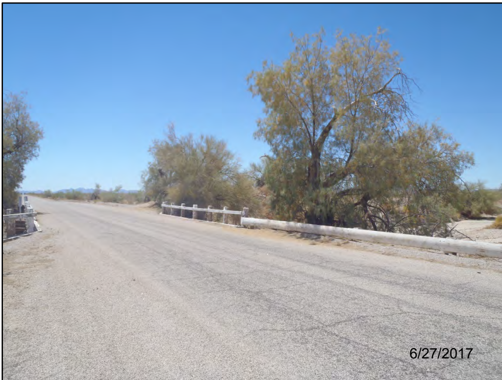
Photo 8. View of Chuckwalla Valley Road adjacent to Sutro Ditch Bridge (#56C0104).
