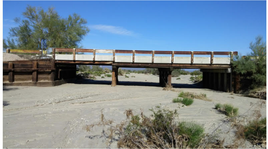
View from Acari Ditch
