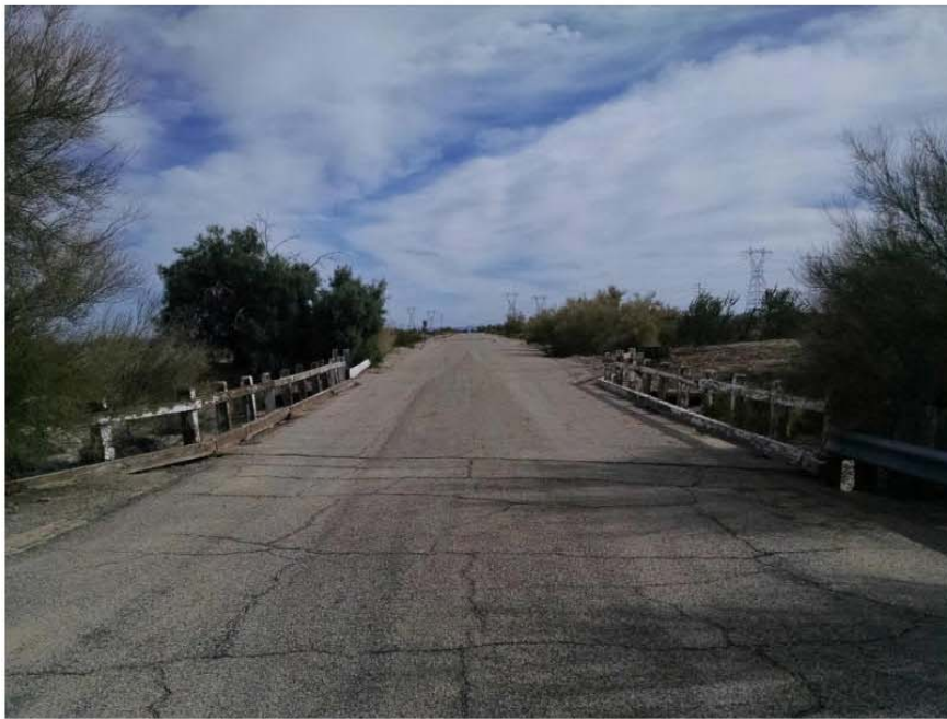
View Approaching Aztec Bridge
