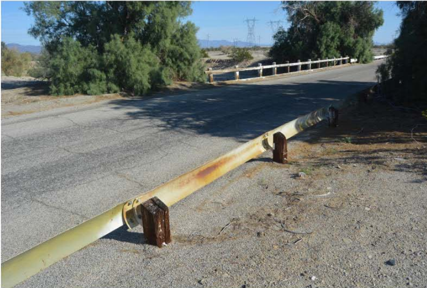
View from Sutro Bridge
