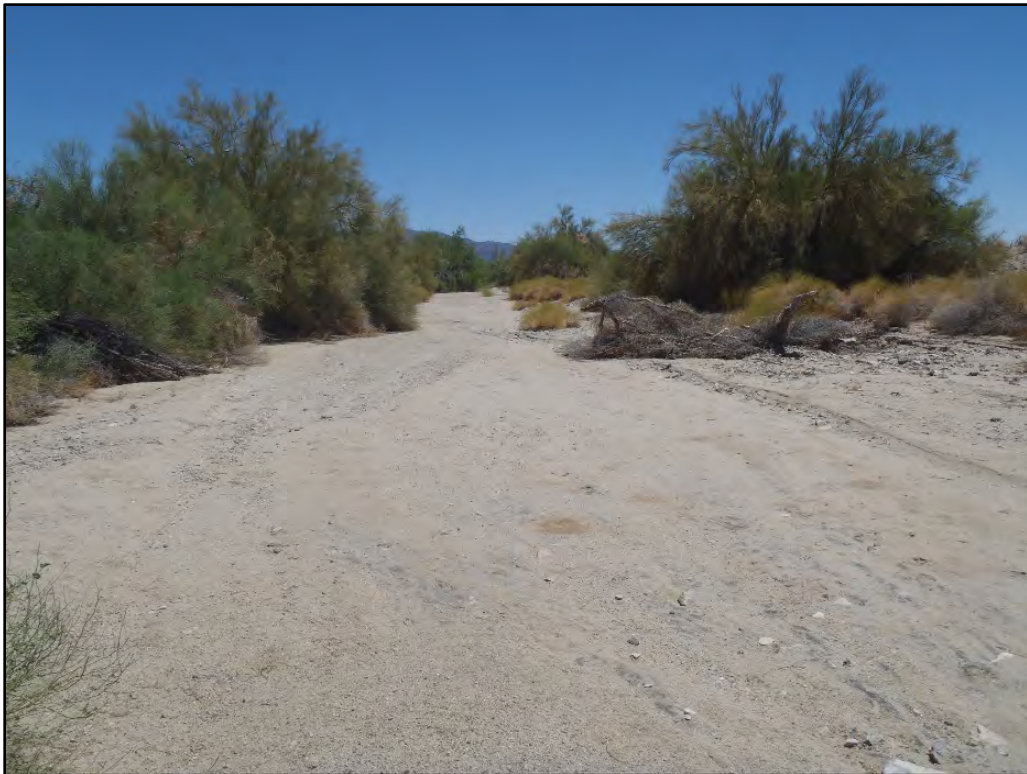
Photo 4. View north from Aztec Ditch Bridge (#56C0102) and the desert wash.
