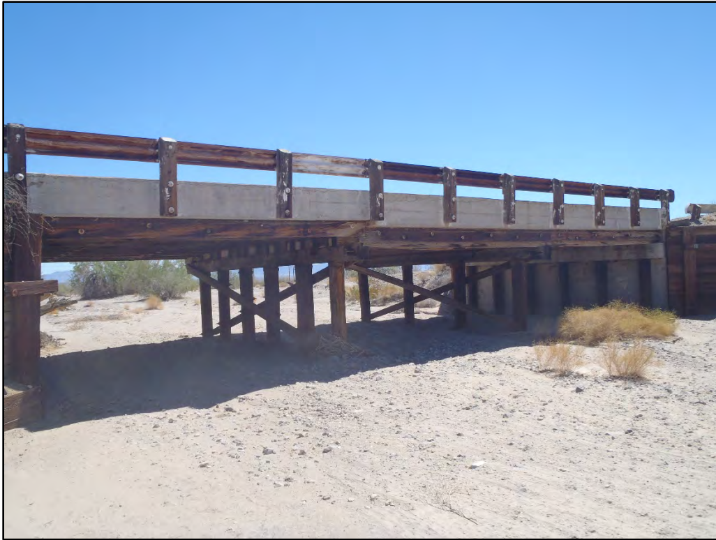
Photo 7. View of Sutro Ditch Bridge (#56C0104).
