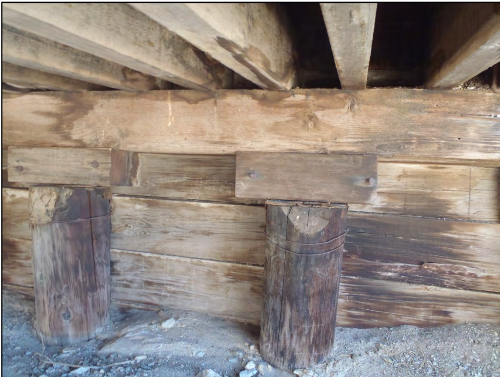
Photo 6. View of existing bridge footings at Tarantula Ditch Bridge (#56C0103).
