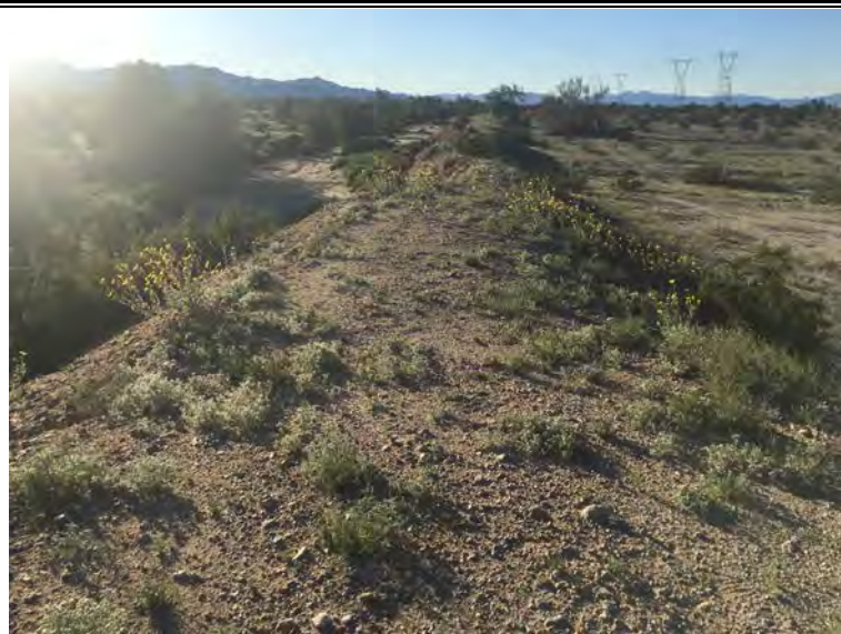
Photograph: 1-17 Photo Date: 02-19-2019 Location: Feature 2-3 Direction: West Comment: View of the man-made diversion dike, taken from the top of the diversion dike along the west side of Feature 2-3.
