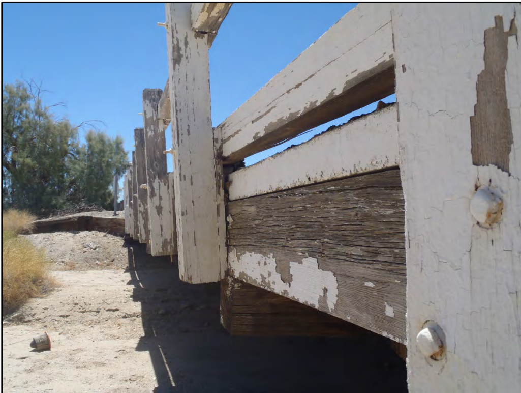
Photo 2. View of the timber bridge at Aztec Ditch.
