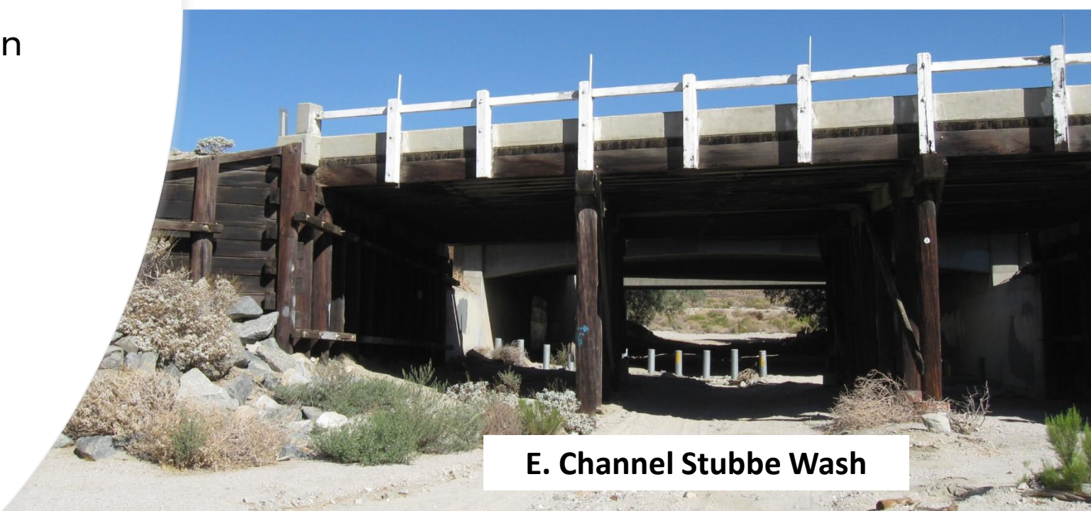
Fornat Wash Bridge
