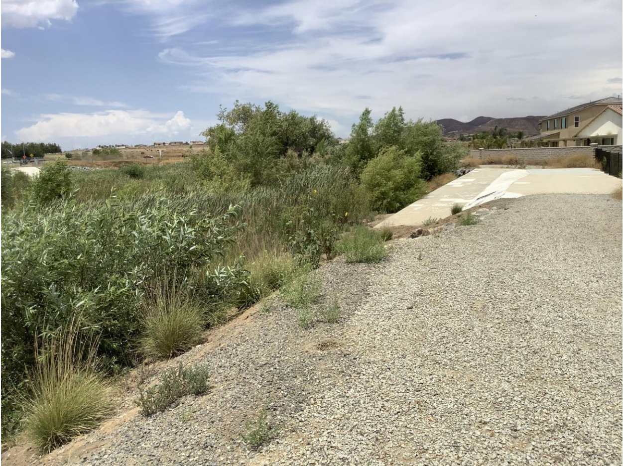
Photo 5: Representative of the slope protection in place separating French Valley Creek from nearby urban development (Taken July 2019).
