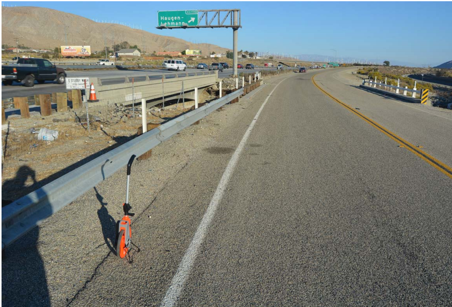
Figure 3. View from Bridge over East Channel Stubbe Wash
