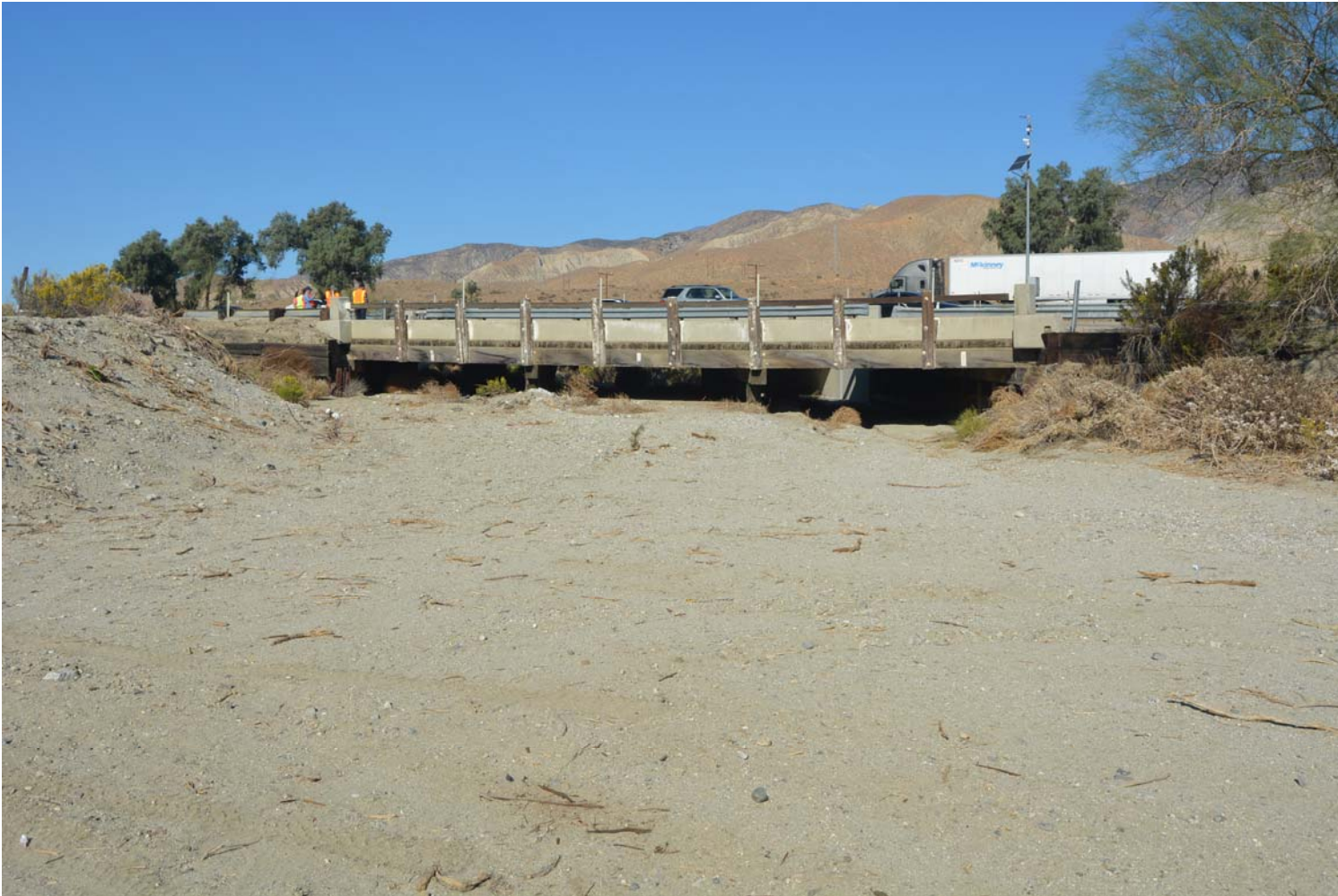
Figure 4. View of the Bridge over Fornat Wash from Ditch
