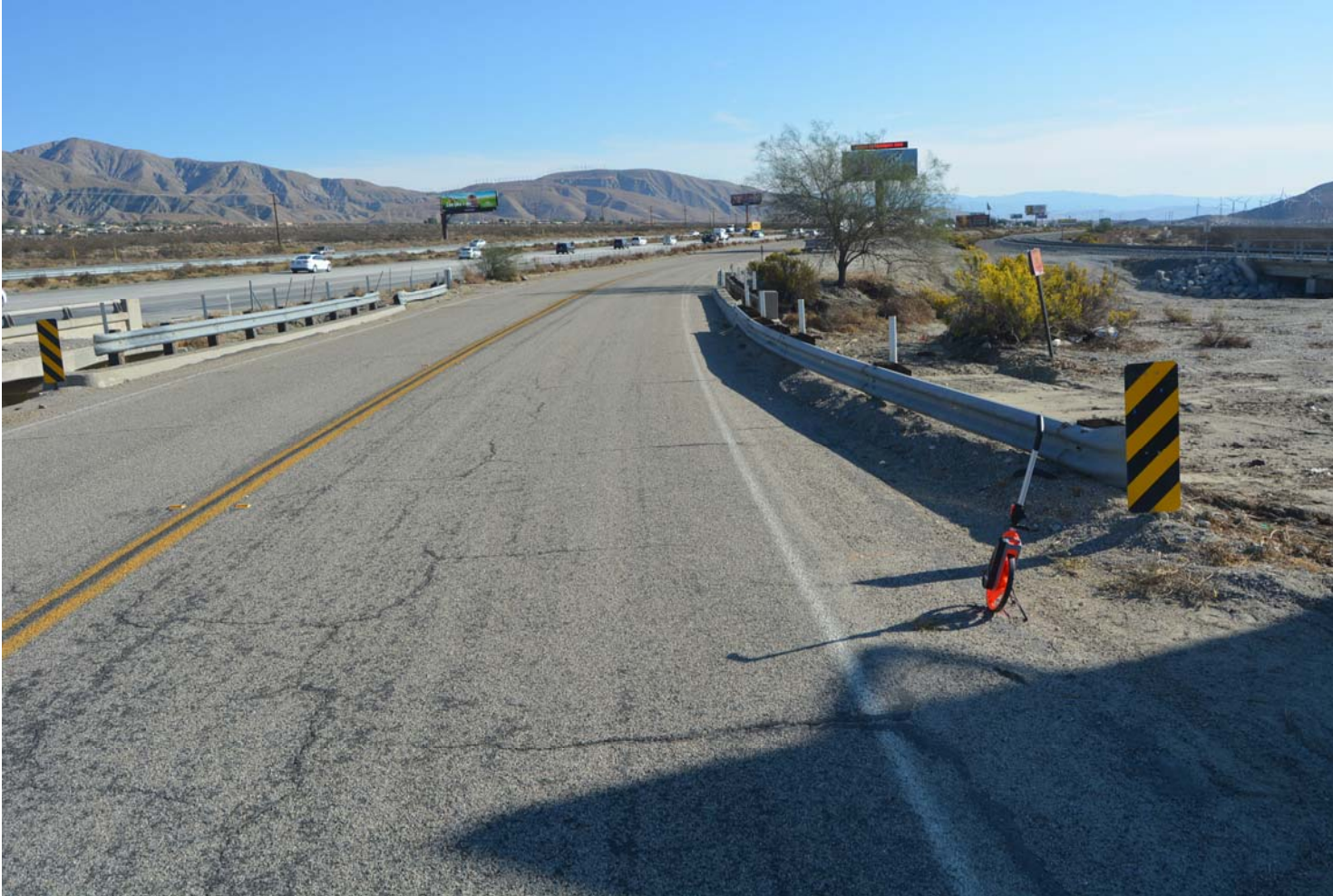
Figure 2. View from Bridge over Fornat Wash
