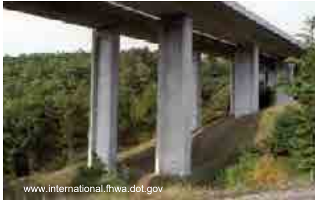
Figure 65. A viaduct in Slovenia built to accommodate wildlife, hydrology, and human connectivity.
