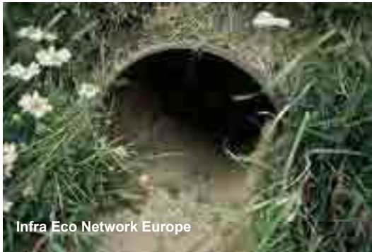
Figure 67. Pipe culvert designed to accommodate small mammals.
