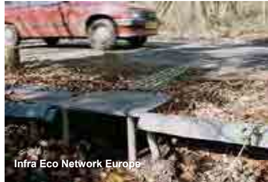
Figure 68. Amphibian tunnels allow light and moisture into the structure.
