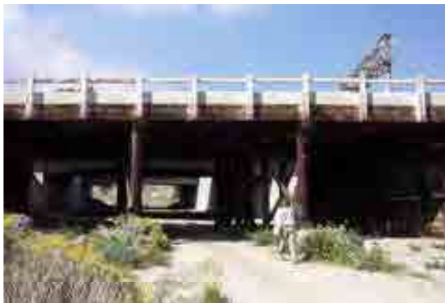
Figure 74. Looking through the easternmost bridges under the freeway and service road.
