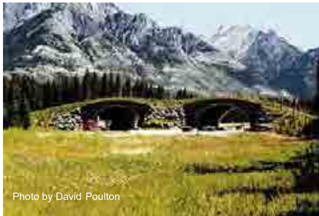
Figure 64. An example of a vegetated land bridge built to enhance movement of wildlife populations.
