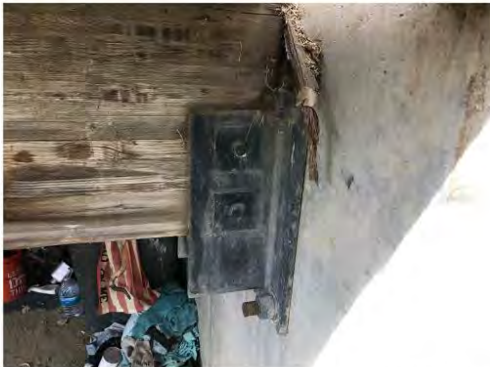
Photo 14: Black (LBP) metal bracket, north abutment, associated with sidewalk support beam (AES XRF Sample: 049).
