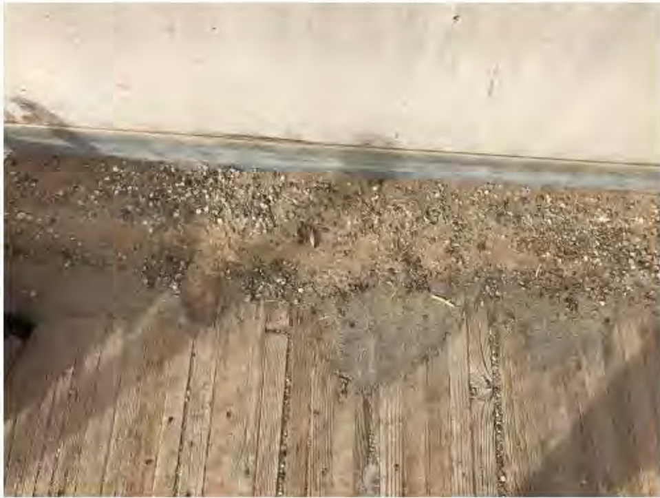
Photo 01: Granular traction coating on upper surface of wood sidewalk (AES Samples: MISC-001-01, 02 & 03).
