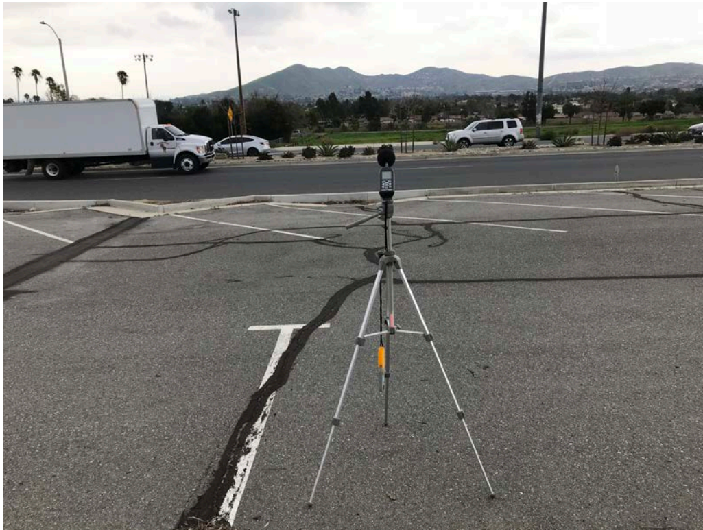
Photograph 13. ST-2 Looking East
