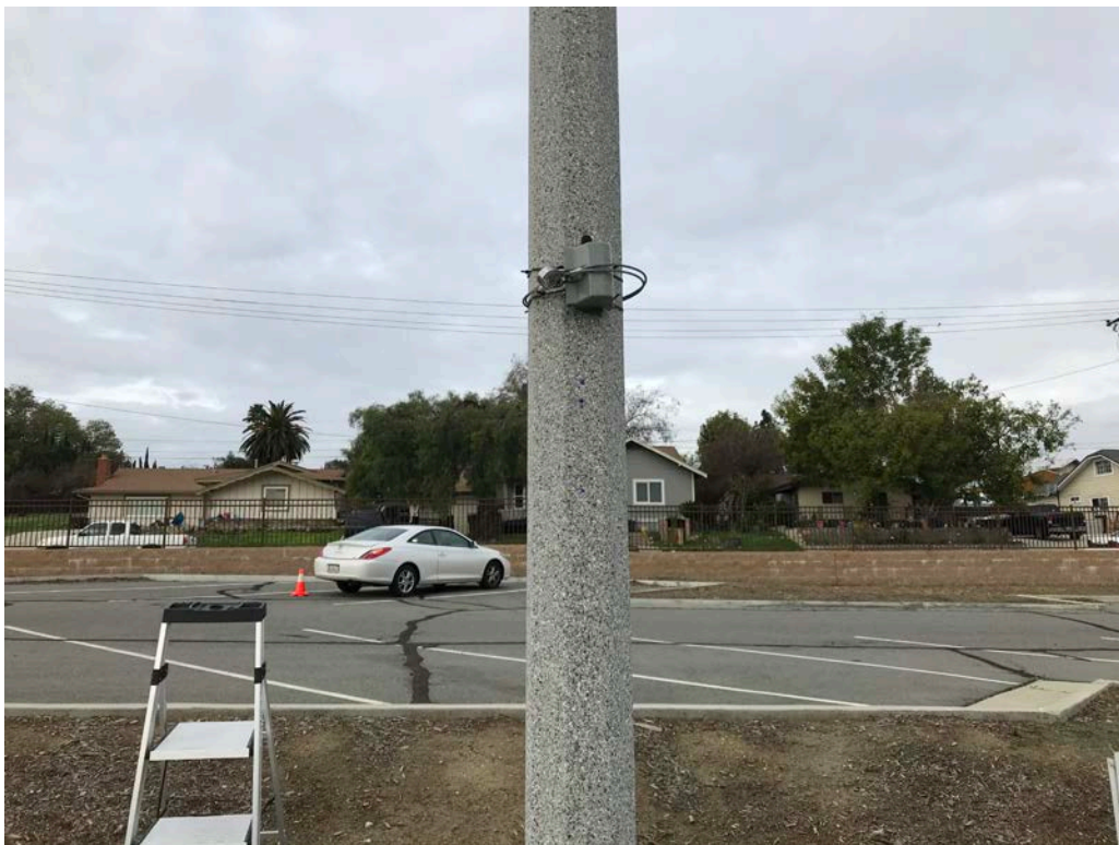
Photograph 4. LT-I Looking West
