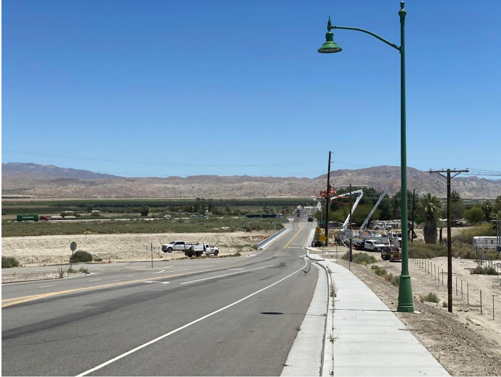
View of Airport Boulevard Bridge facing East showing utility poles, barren soils, and new yellow striping along Airport Boulevard (October 2020).
