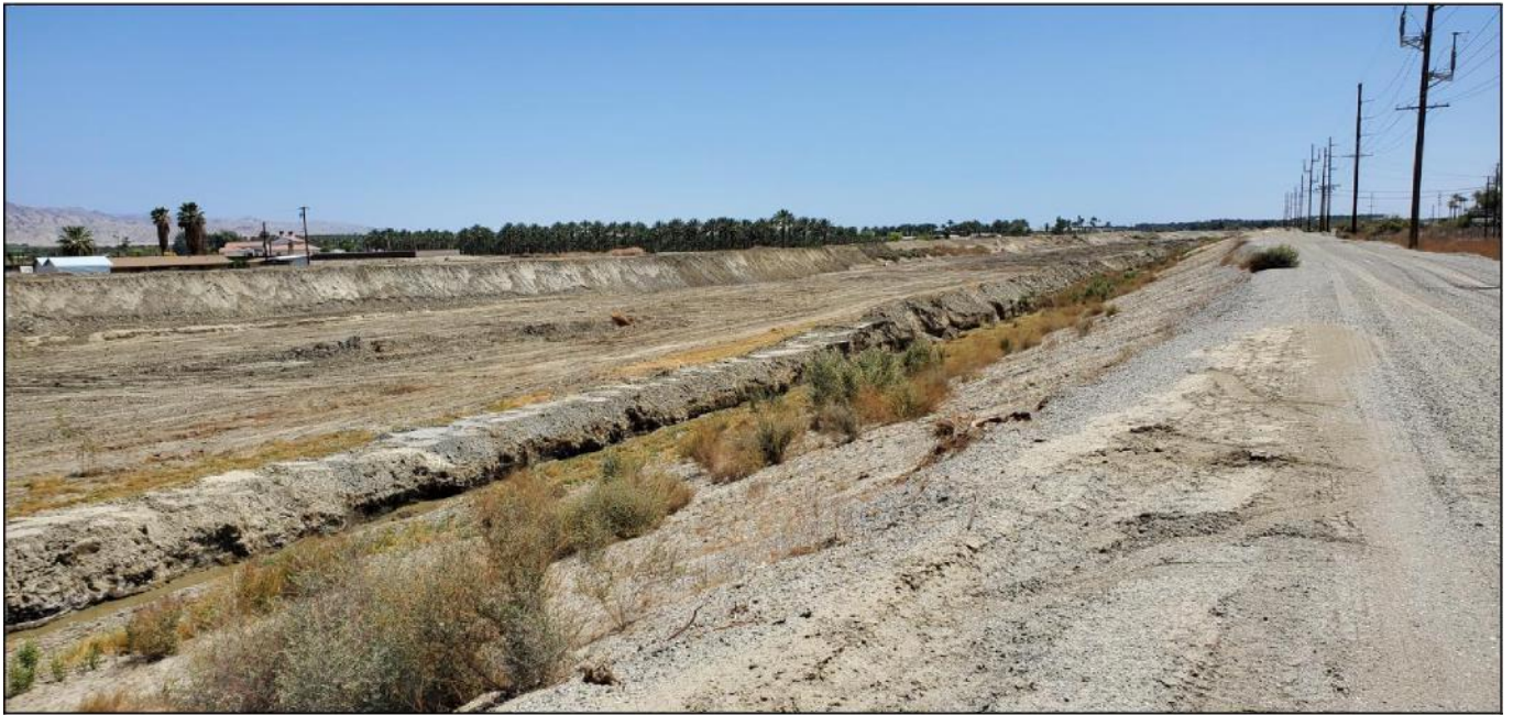
Figure 5. Overview of southern end of the project area
