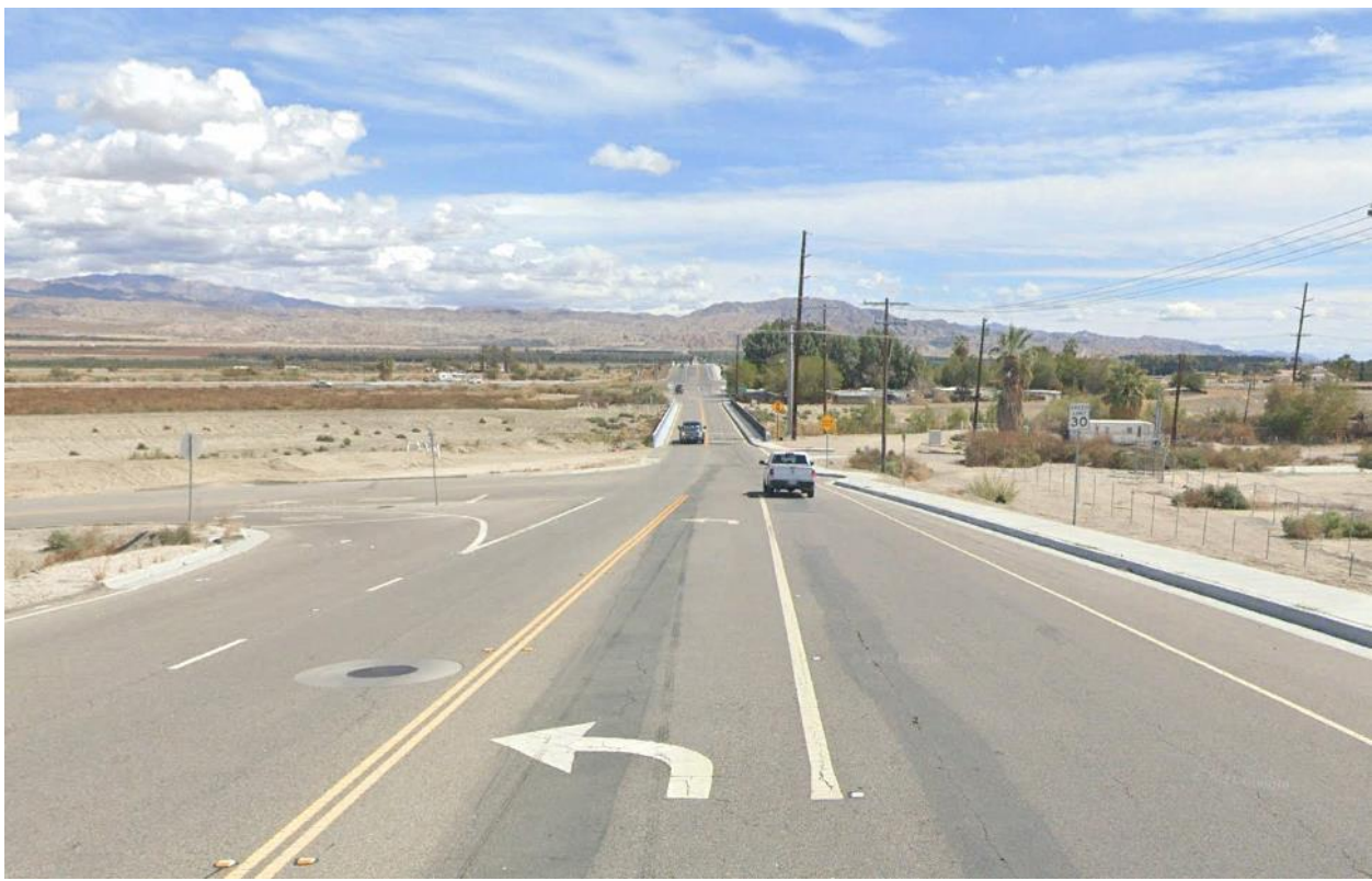
Photo 1: Looking east on Airport Boulevard 400 feet west of the intersection of Airport Boulevard and Orange Street in the Thermal Area. This view is representative to motorists along Airport Boulevard. Image taken November 2018.
